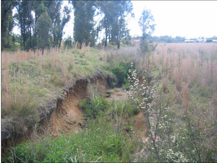
Figure 14. Drainage channel in Survey Unit 3.
